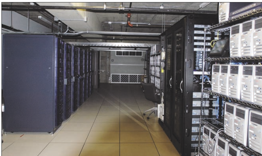
The planetarium's computer room features a Silicon Graphics supercomputer (left) and computers for networking and storage.
